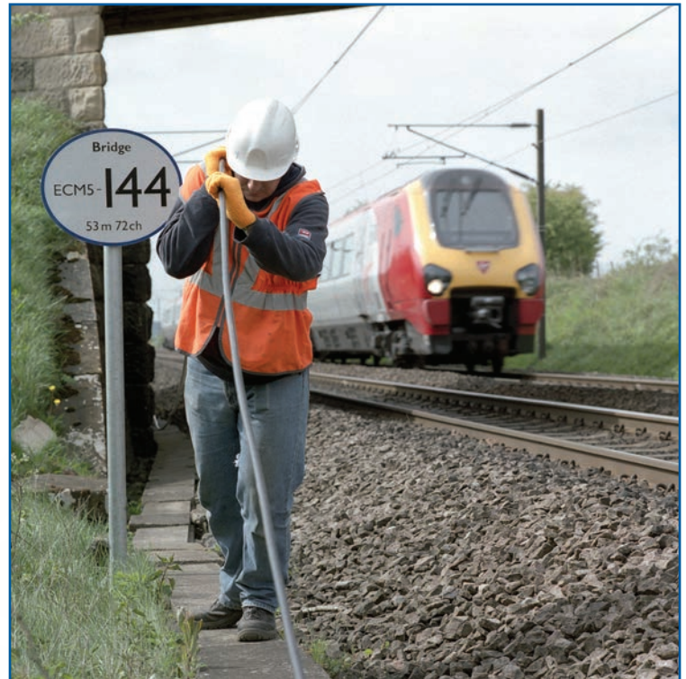
Telecommunications installation by Skanska for Network Rail
